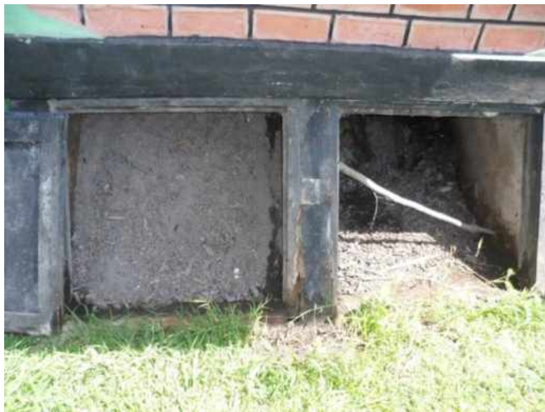
The left vault is full and needs emptying.
